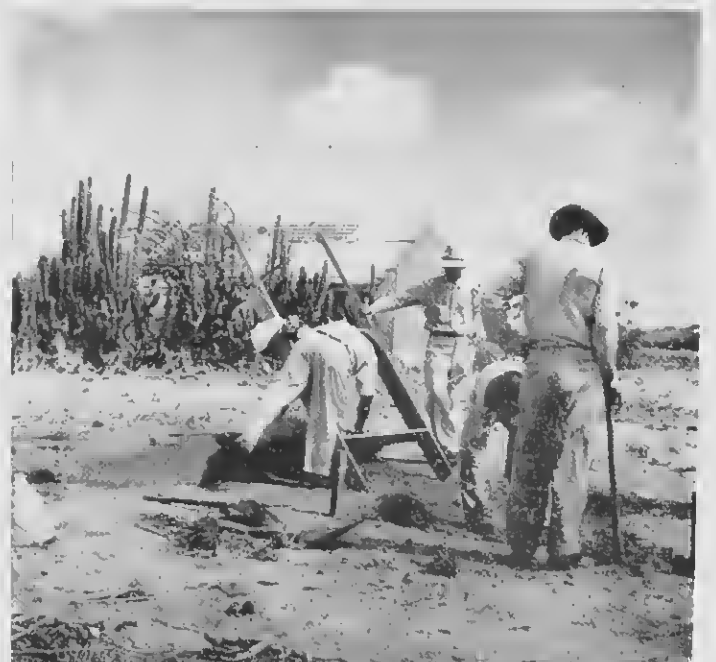
PUBLIC WORKS team, digging near surface on Arends farm.
